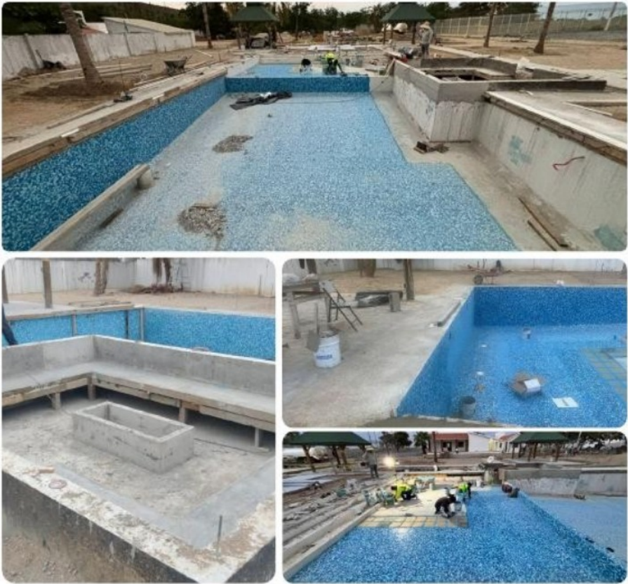
Alberta Closter Project | Puerto Balleto, Islas Marías | 2024 The solution combines concrete, wet-area coatings, non-slip pavements, and stone aggregates selected for strength, low maintenance, and adaptation to the coastal environment.
